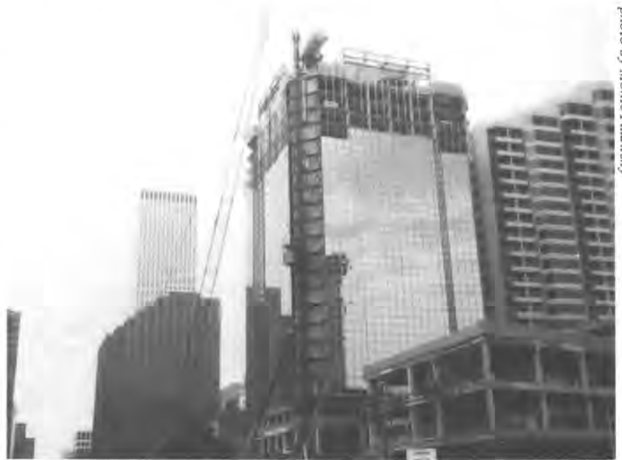
THE CITY'S CURRENT BUILDING BOOM
