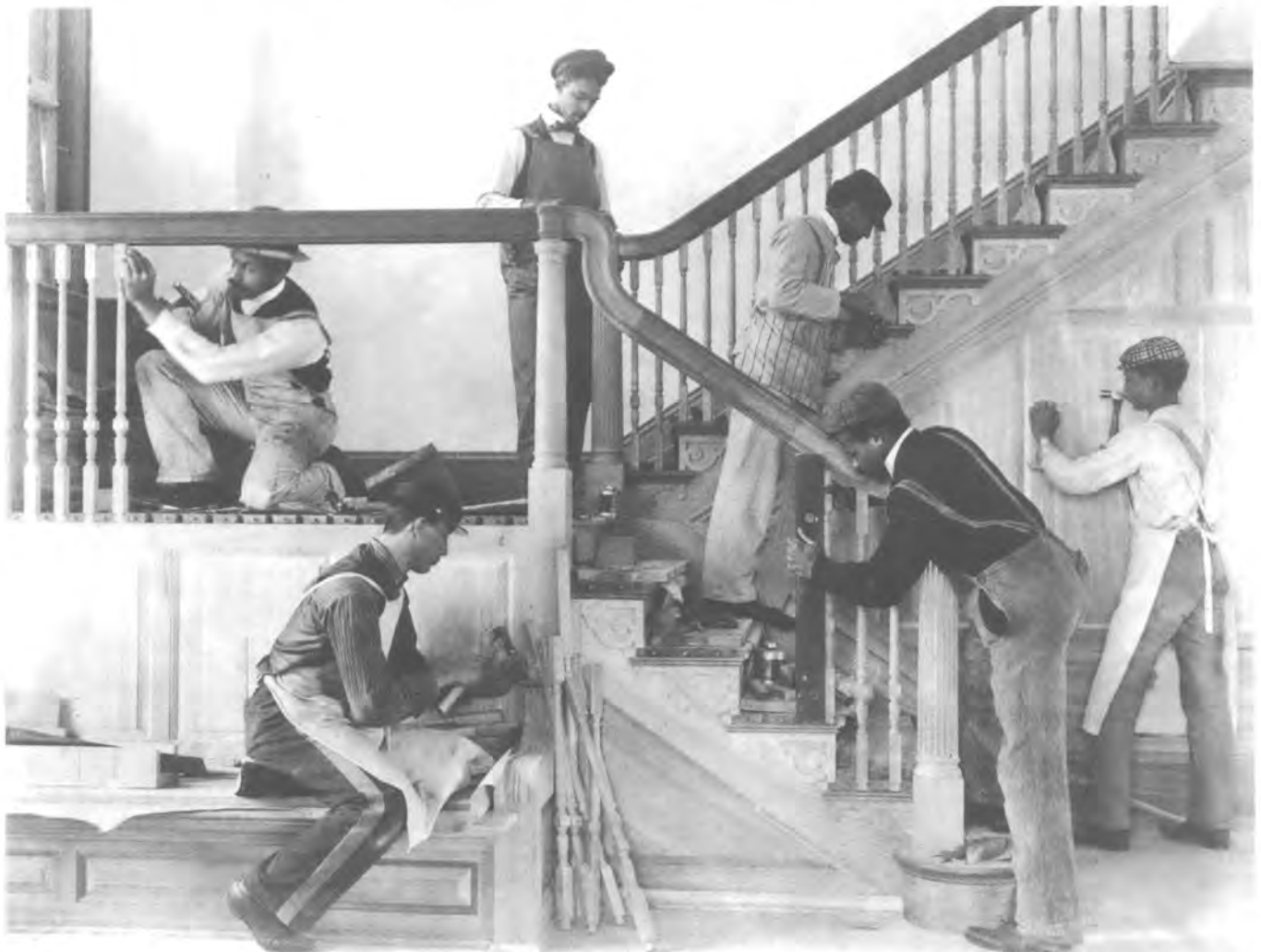
BELOW: "STUDENTS BUILDING STAIRWAY OF HOUSE, HAMPTON INSTITUTE," BY F.B. JOHNSTON, 1899.
