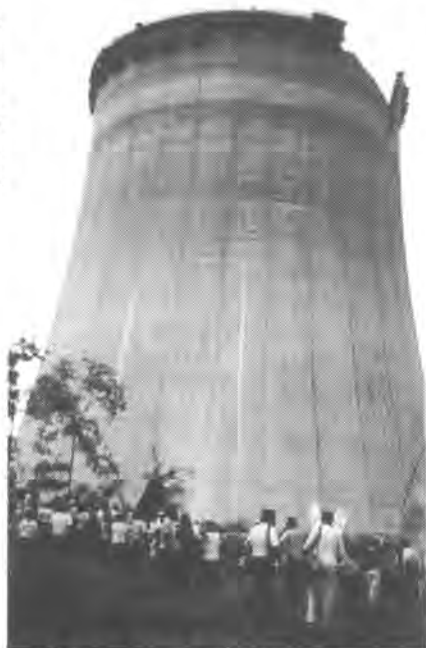
DEMONSTRATION AT GRAND GULF DURING CONSTRUCTION. NOTE TORNADO-DAMAGED COOLING TOWER.
