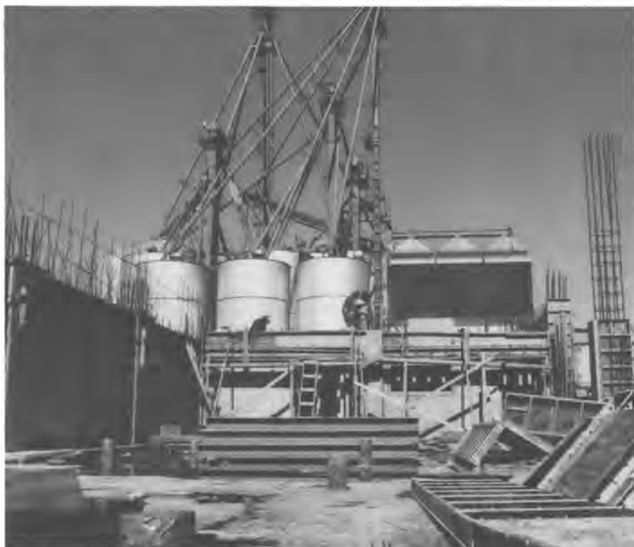
Grain elevators rise above construction of farmer-owned flour mill in Dawn.
