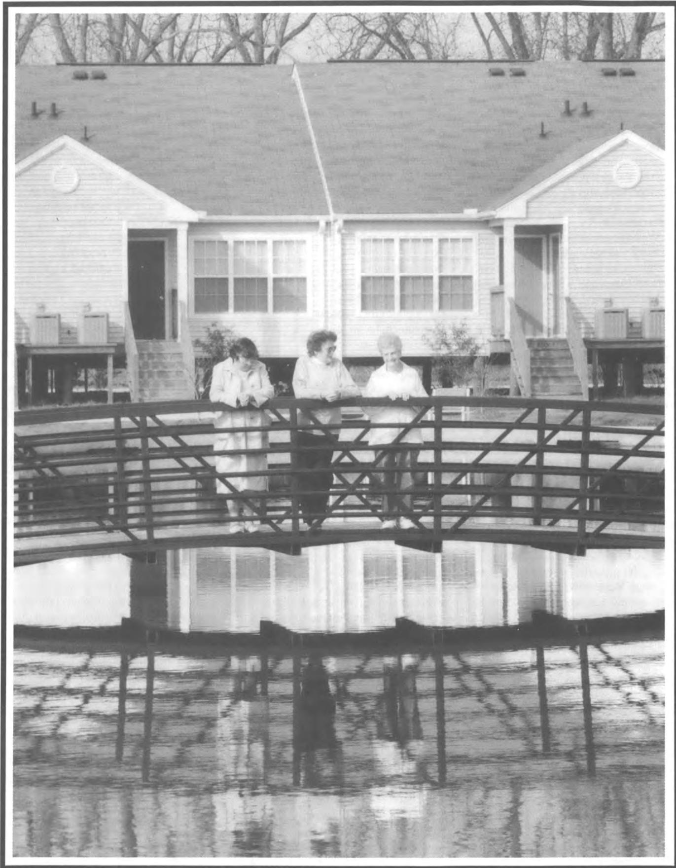
THE TOWN OF BELHAVEN, NORTH CAROLINA CREATED PUNGO VILLAGE, A COMPLEX OF 38 APARTMENTS FOR THE ELDERLY BUILT AROUND A LAKE.
