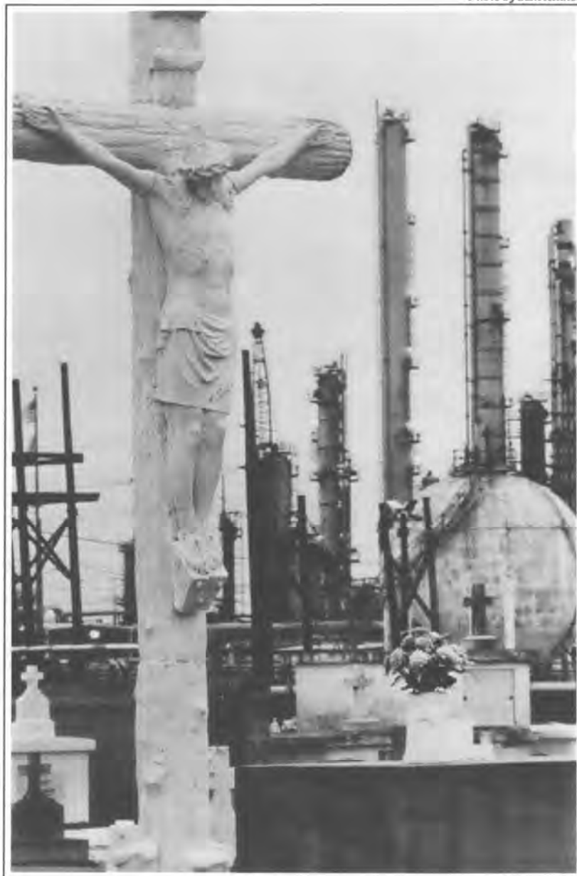
A TANK CAR EXPLOSION AT THIS UNION CARBIDE PLANT IN TAFT, LOUISIANA FORCED THE EVACUATION OF 18,000 PEOPLE IN 1985. RESIDENTS IN A NEARBY HOUSING PROJECT COMPLAIN OF EYE, MOUTH AND NOSE IRRITATION, AND THE EPA SAYS NEIGHBORS FACE CANCER RISKS AS HIGH AS 1-IN-100 FROM THE PLANT'S ETHYLENE OXIDE.
