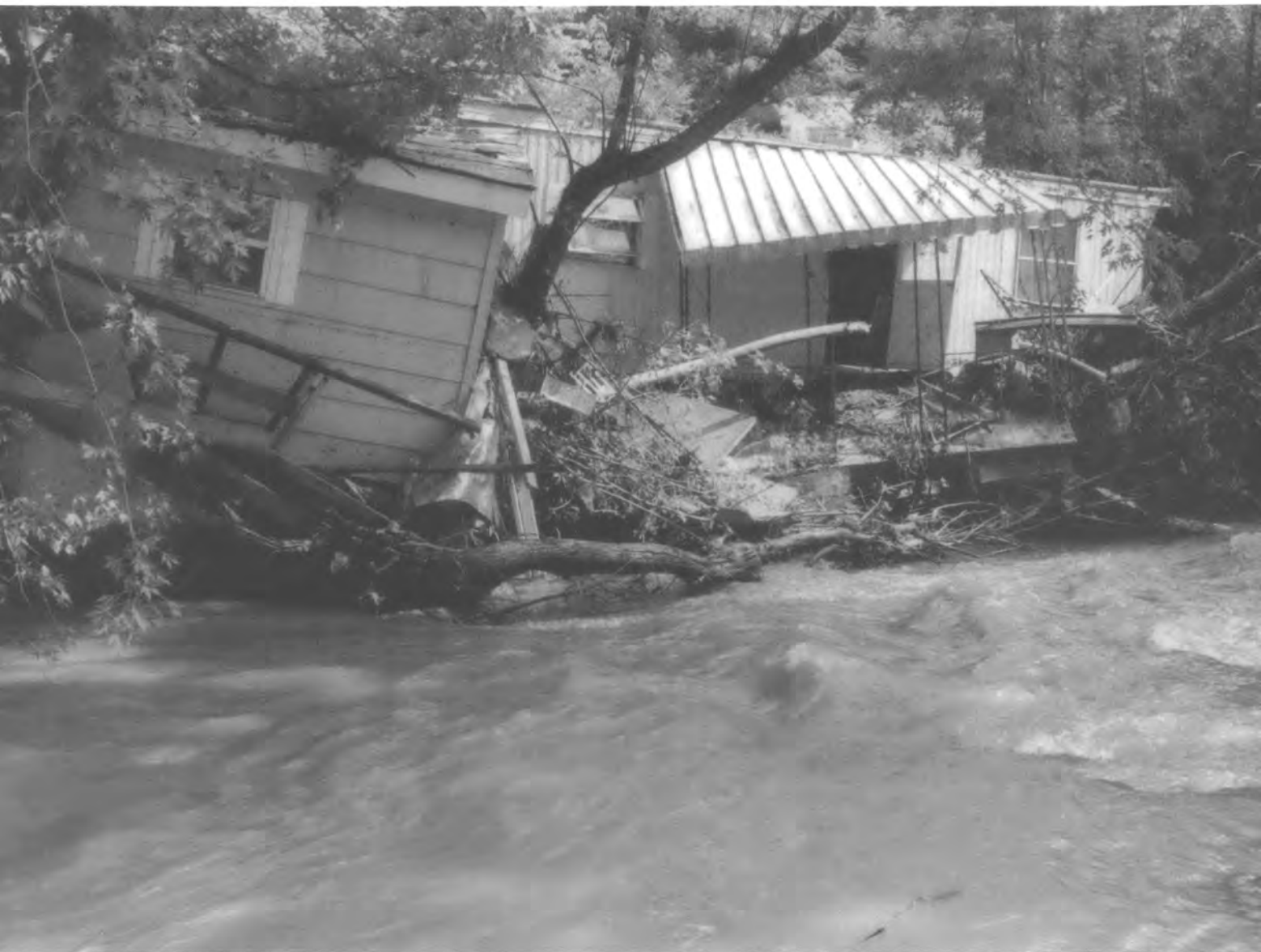
Homes washed into the river in Anawalt, July 2001.
