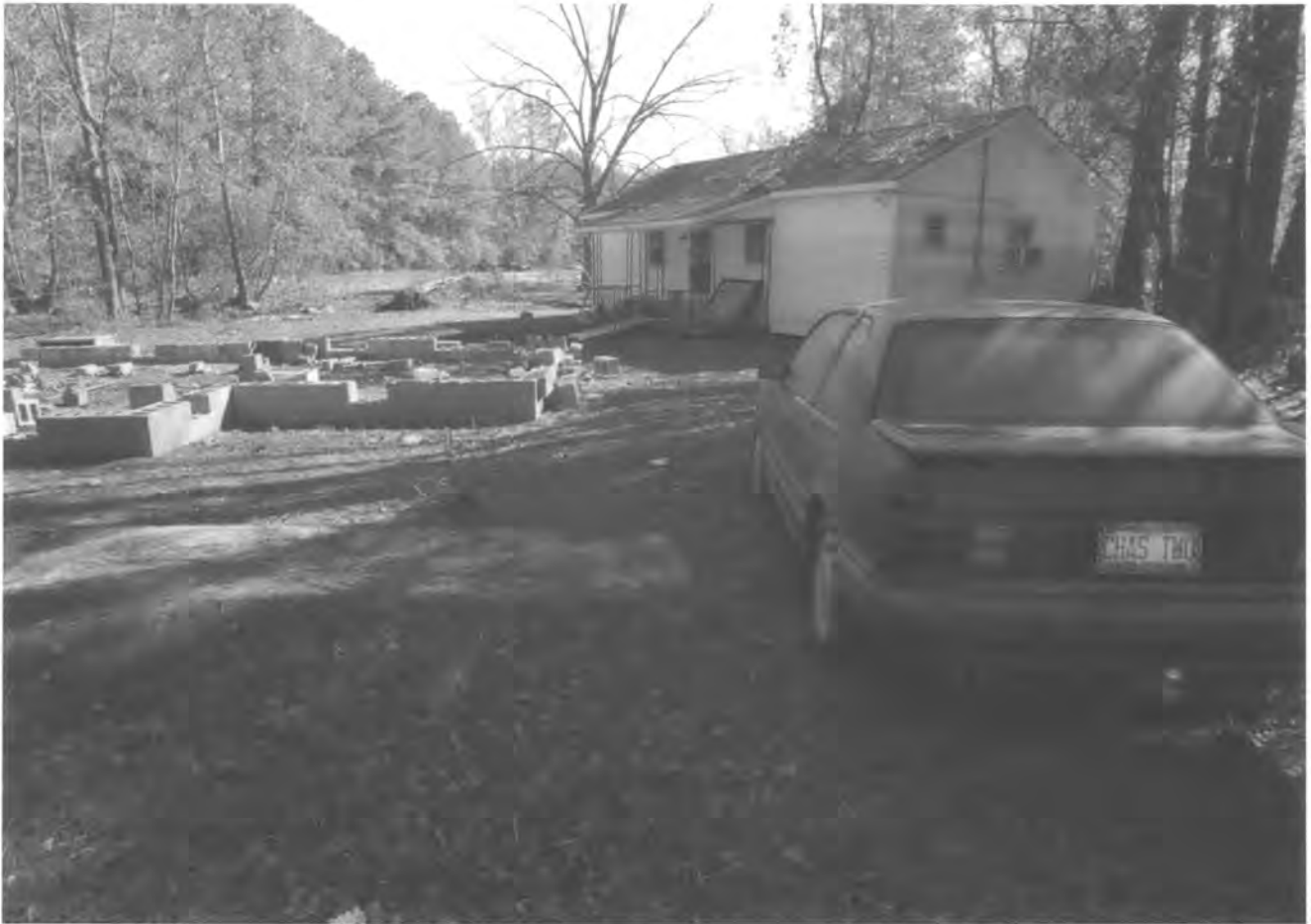
A house in the low-lying section of Princeville that was inundated by Hurricane Floyd in 1999. Photo: Hart Matthews
