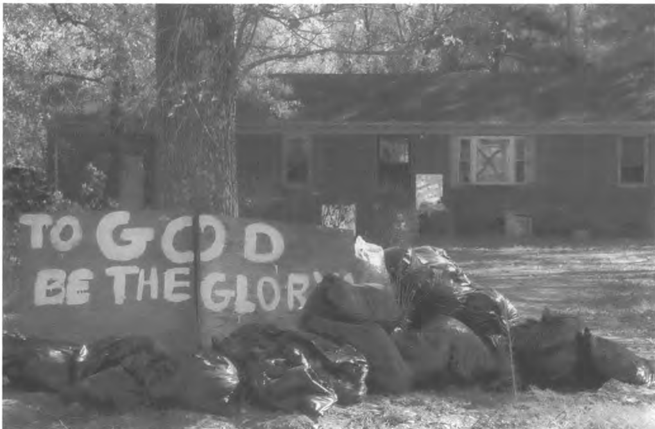
A house in the low-lying section of Princeville that was inundated by Hurricane Floyd in 1999. Photo: Hart Matthews
