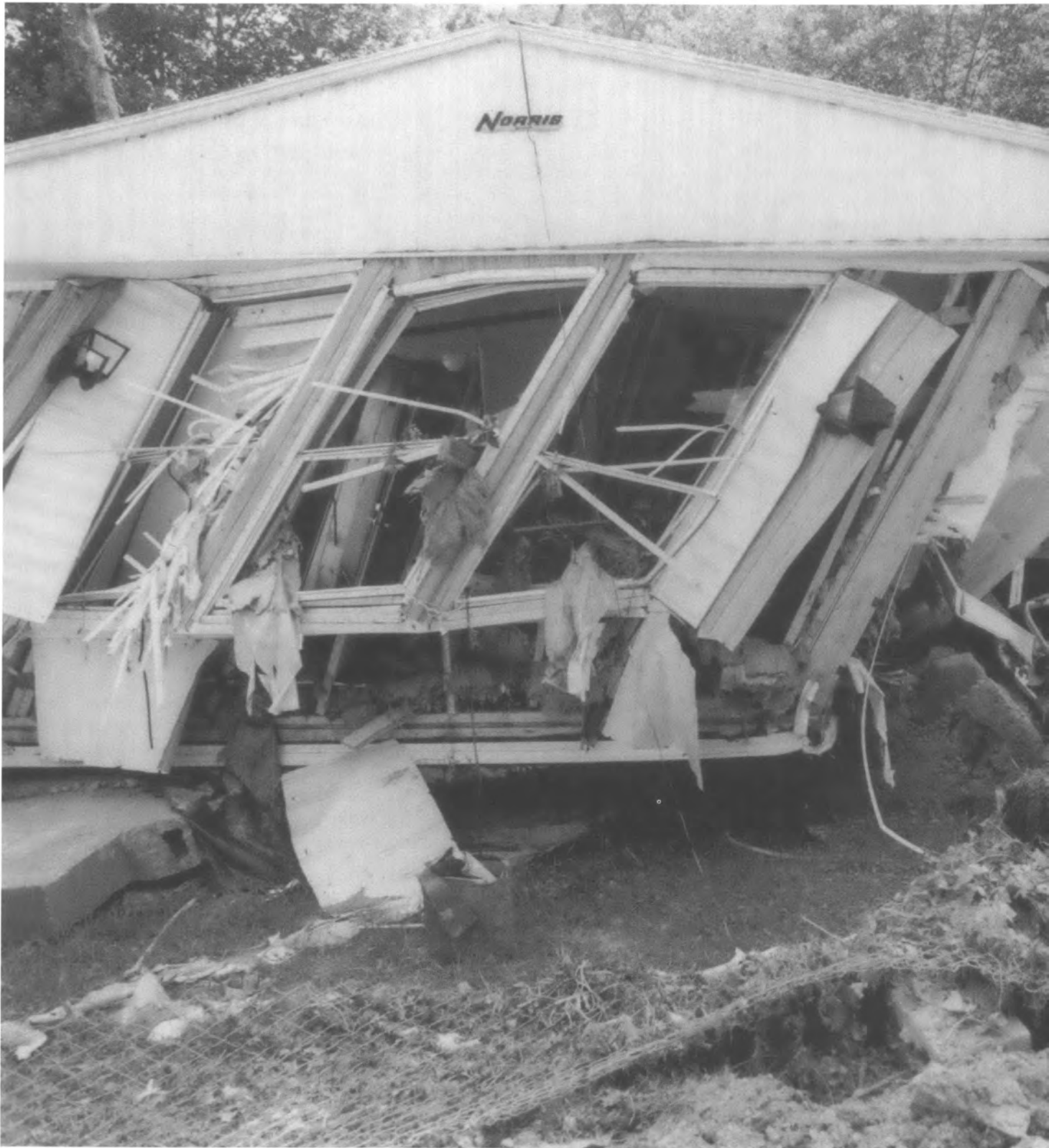
Wrecked homes near Pineville.
