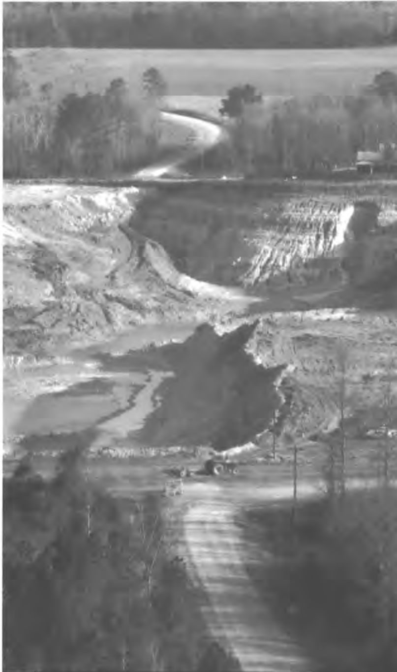
COUNTY OFFICIALS LET KAOLIN MINERS RIP UP OLD HIGHWAY 85 IN DEEPSTEP, GEORGIA AND REROUTE TRAFFIC HALF A MILE AROUND THE PIT.
