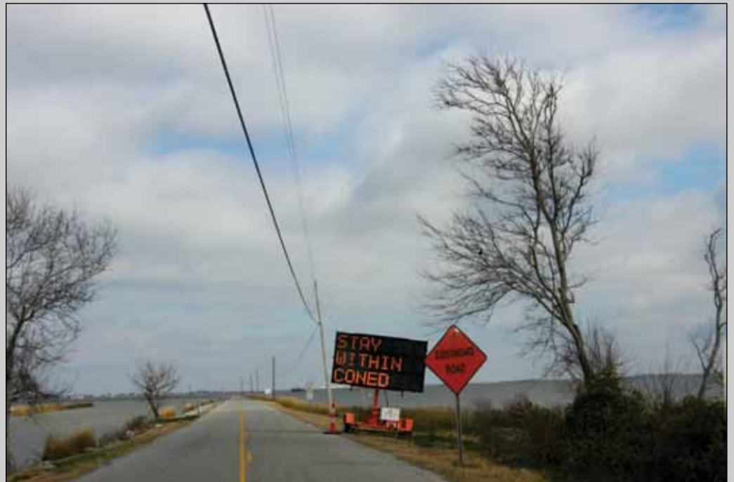
Rapid erosion of the Louisiana coast, which has been accelerated by pipelines cutting through sensitive wetlands, has caused water to steadily encroach on many coastal communities. This road to Isle de Jean Charles, a ridge of land in Terrebonne Parish and home to members of the Biloxi-Chitimacha-Choctaw tribe, must be continually reinforced as the water threatens to overtake it. (Photo by Alysha Jordan)
